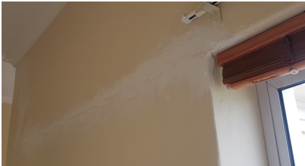
Photograph 8 - Repair work to typical cracks
