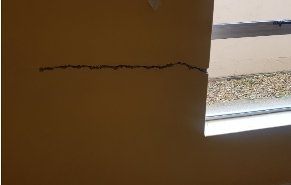
Photograph 9 - Repair work to cracks
