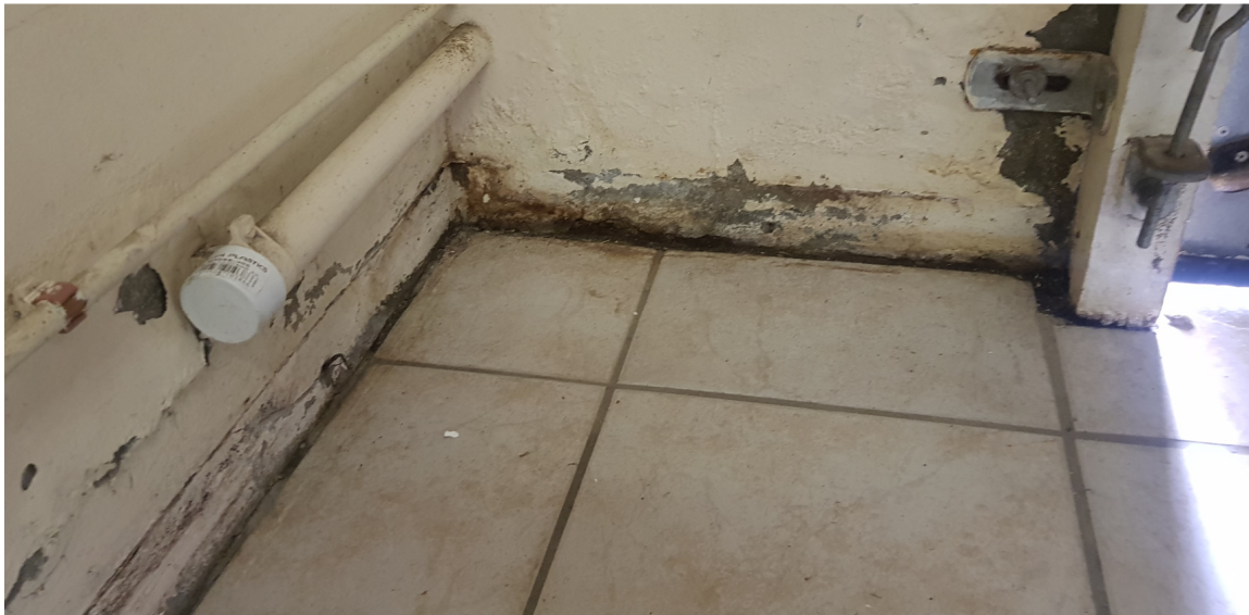
Photograph 3 - Garage wall, adjacent to bathroom
