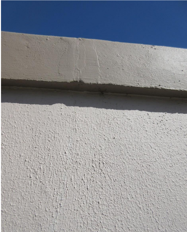
Evidence of moisture causing the paint surface to delaminate; evidence of cracks; evidence of poor repair work to the plaster band at the top of the wall.
