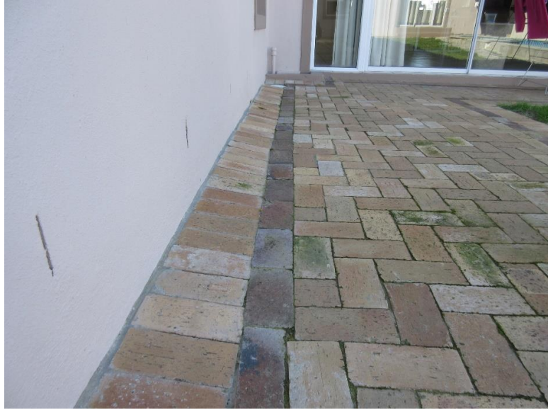
The header course against the wall is completely out of level; no proper grouting to the remainder of the brick paving.
