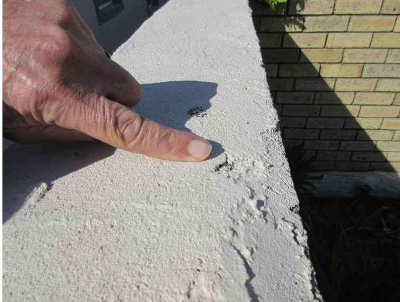
Evidence of very poor quality workmanship on top of this wall.
