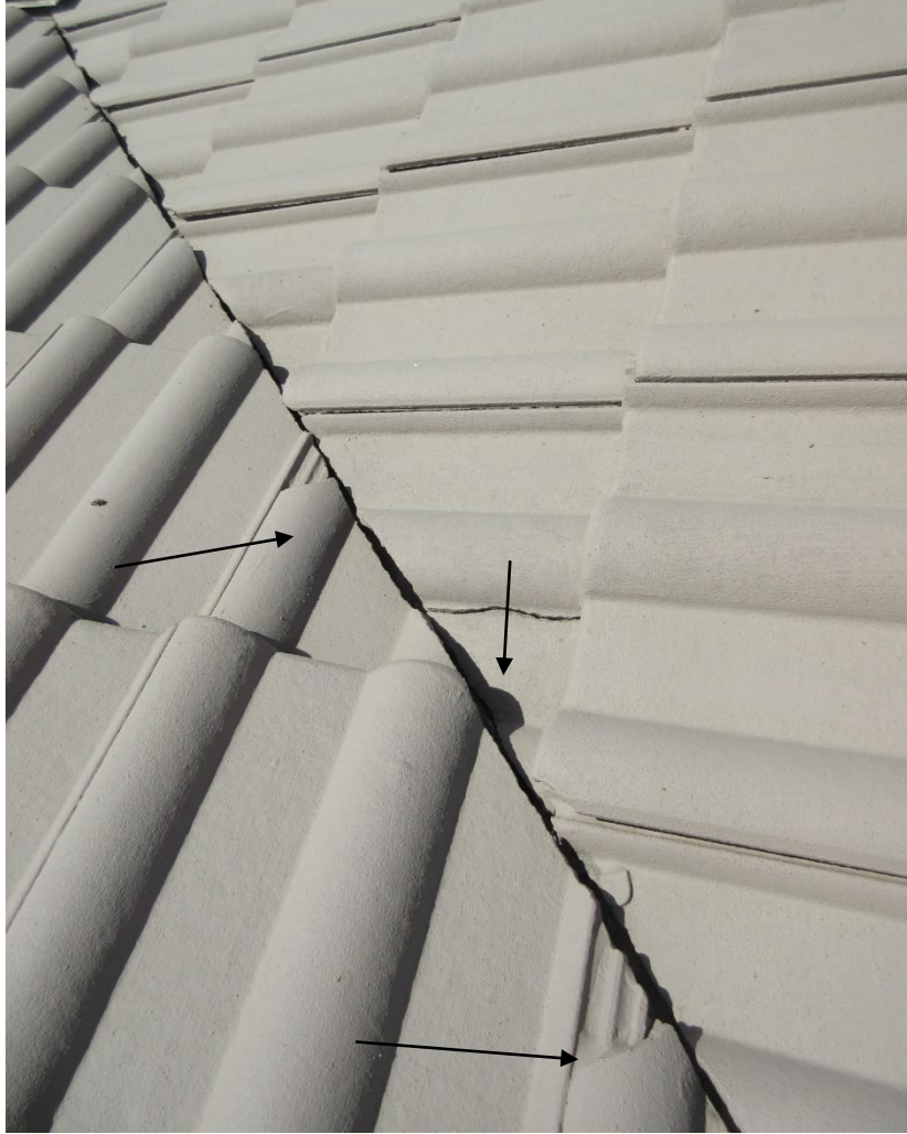
More cracked and broken tiles that have simply been painted over.
