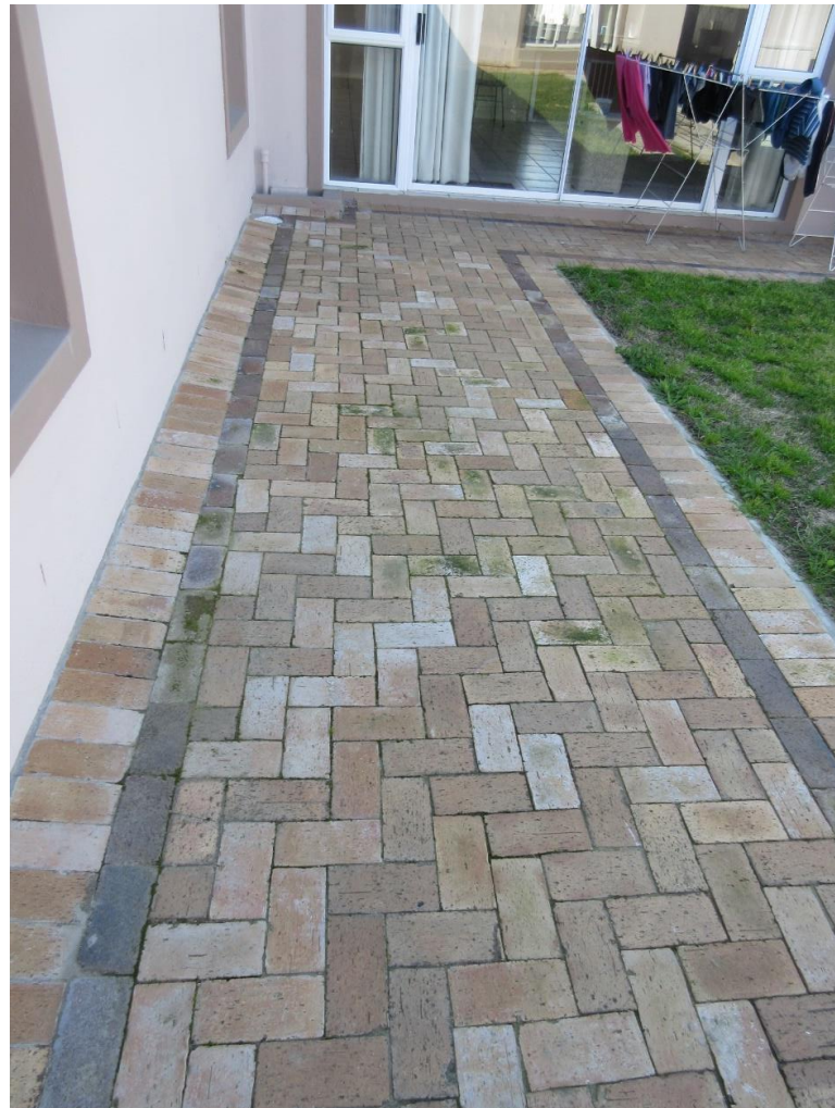
The header course against the wall is completely out of level; no proper grouting to the remainder of the brick paving.
