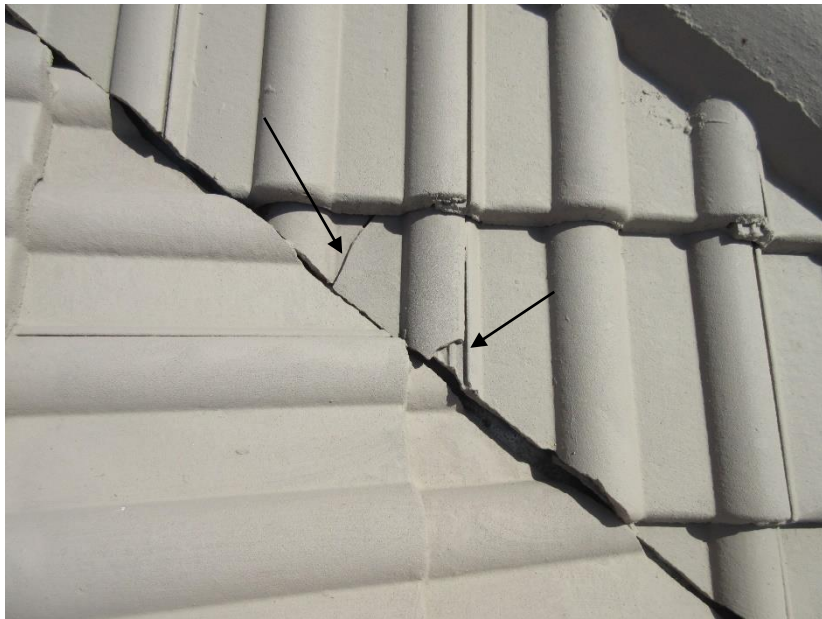
More cracked and broken tiles that have simply been painted over.
