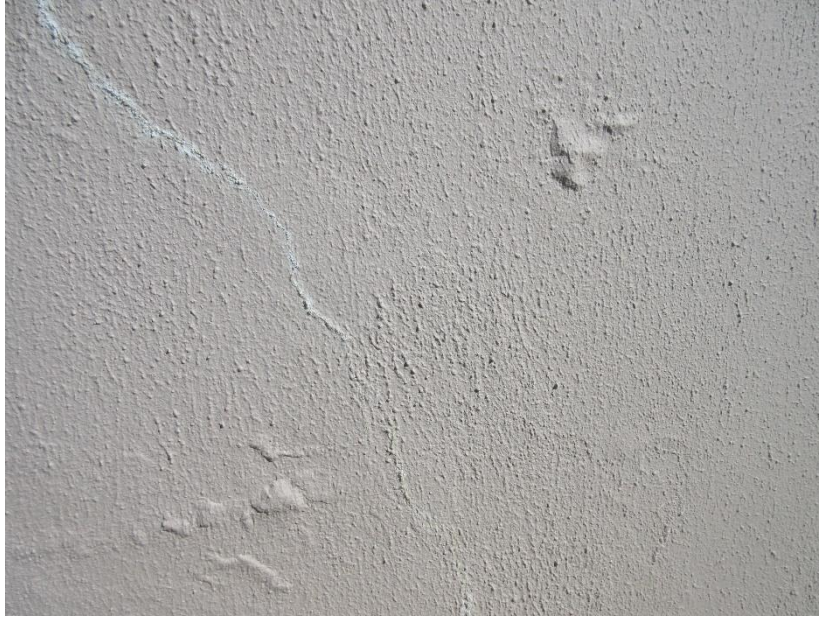
Evidence of moisture causing the paint surface to delaminate; evidence of cracks; evidence of poor repair work to the plaster band at the top of the wall.
