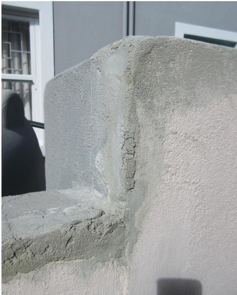
Further evidence of very poor quality and inferior plaster work.
